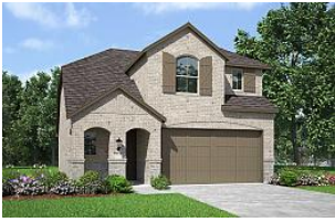
306 Highland Bayou Drive
